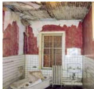
**THREAT:** The building is in need of immediate repair to address moisture intrusion and deteriorating masonry.
