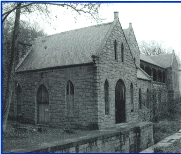
Byrd Park Pump House
